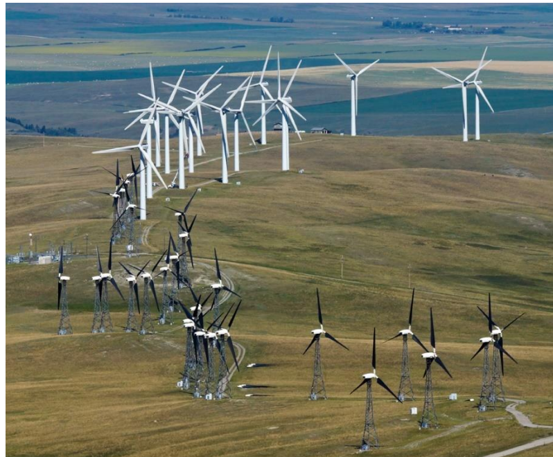
Pincher Creek area wind farms – Clive Schaupmeyer
